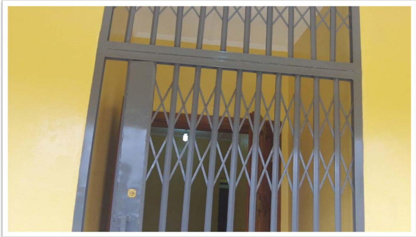
SLIDE 4. Accordion Steel Gate At The Main Entrance To The Kahnplay Magisterial Court Building.
