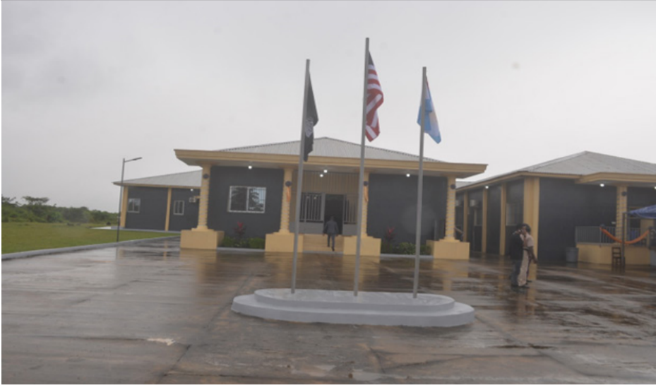
Judiciary Branch of Government Dedicates State-of-the-Art 14th Judicial Circuit Court Complex...to enhance Infrastructure Development in the Judiciary & Promote Access to Justice
